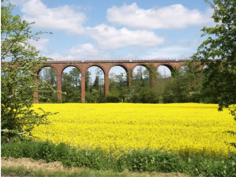
Part of the 30 arch viaduct seen across the meadows of the River Leadon.
