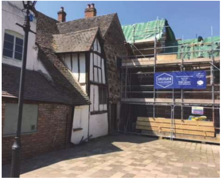
31 High Street undergoing renovation
